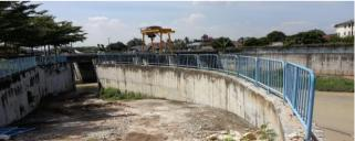
Part of flood mitigation plan for Kuala Lumpur city centre is to reduce Sq. Gombak flow into the city. This was done by bypassing the flow towards Batu Pond by construction of Sg. Gombak bypass and a barrage to control the flow at the intake. The barrage is operated by Department of Irrigation and Drainage Malaysia.
